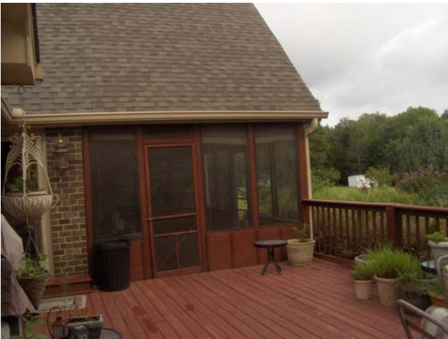
<screened in patio
